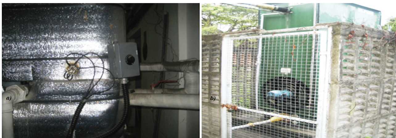
Figure 3. a) Electric resistor set and chilled water tank. b) Cooling Tower – Cold water circuit.
