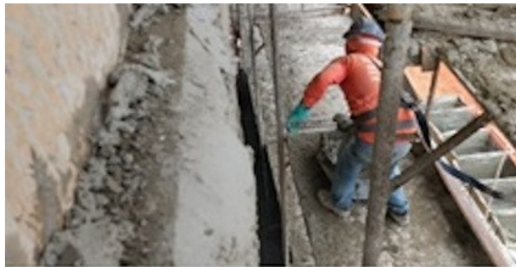
Figure 3. Outside plaster on scaffolding facade.
