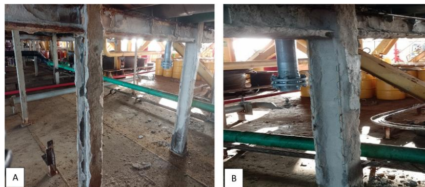
Figure 8. Spraying of mortar for passive protection.
