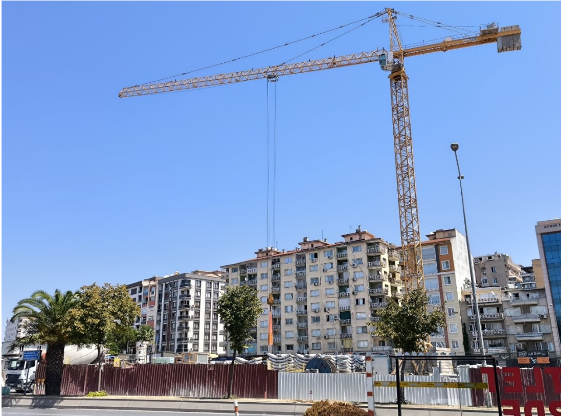
Figure 1. Tower crane in building construction.
