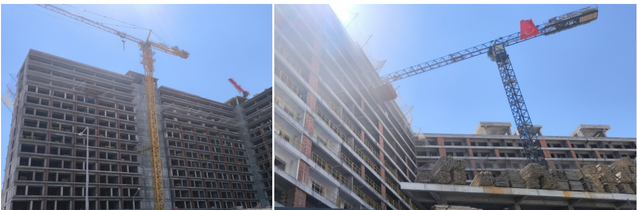
Figure 2. Installed tower cranes in different building areas.
