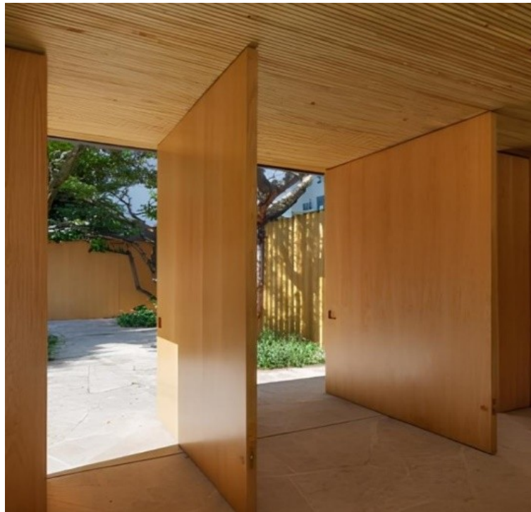
Figure 2. Slab of NLT - Caconde Source: Rewood – Structural Timber Solutions ( https://rewood.com.br ), accessed in 2021.
