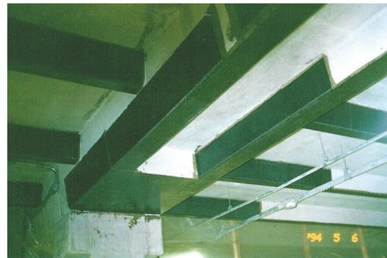
b) bonding of CFRP
