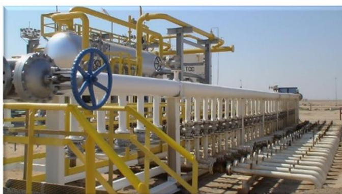
Figura 5. ‘Manifold’ (Oil Wells Manifold (2021)).
