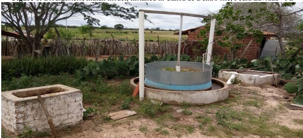
Figure 6: Biodigesters, Indian model, installed in Canoa de Dentro site, Pedra Lavrada - PB
