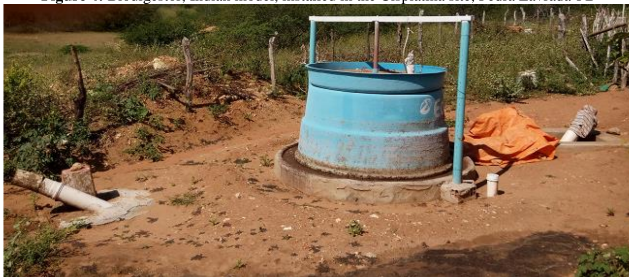
Figure 4: Biodigester, Indian model, installed in the Cisplatina site, Pedra Lavrada-PB
